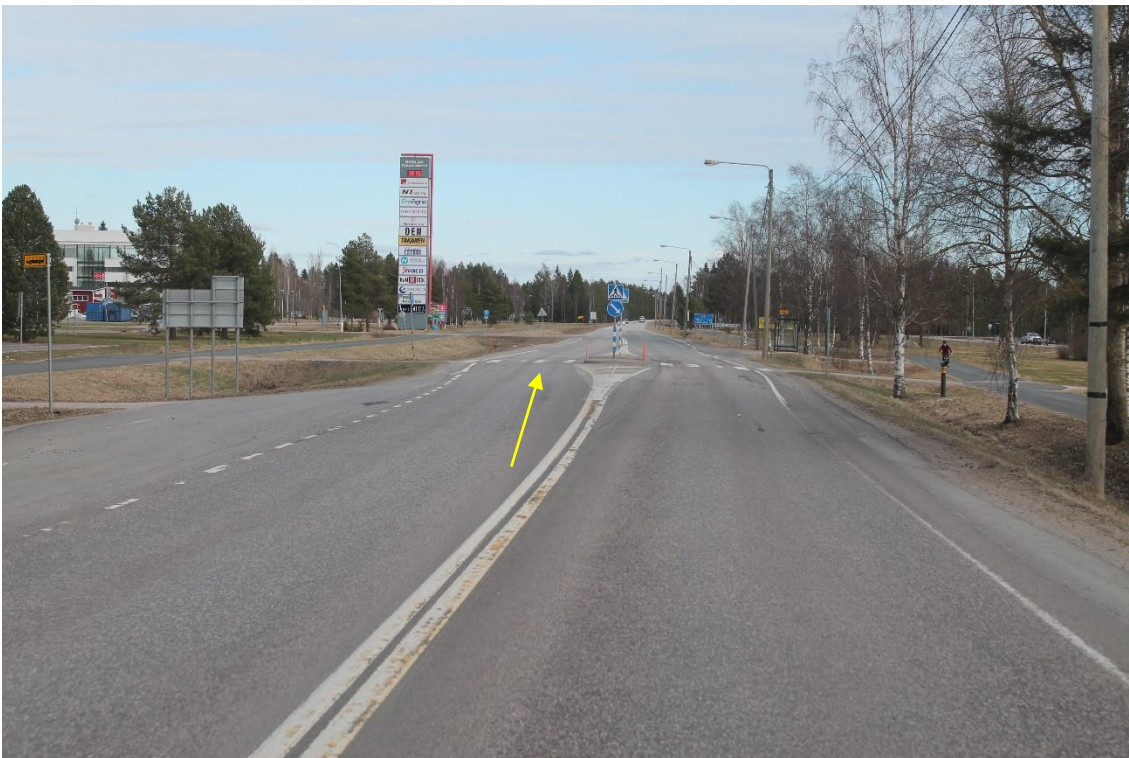
Pos 17/Pic 26. Road 27 in Nivala. https://goo.gl/maps/7V5XxLvcW9r4u68t7 Need to use counter lane or signs need to be removed.
