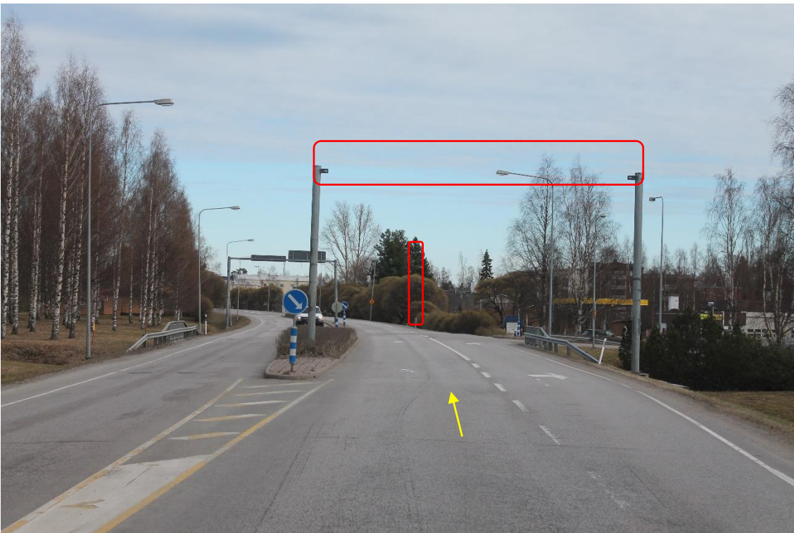
Pos 19/Pic 28. Road 27 in Haapajärvi. https://goo.gl/maps/SgsxkaJi9RDHvih79 Marked portal (missing) and lamp post (missing) need to be removed.
