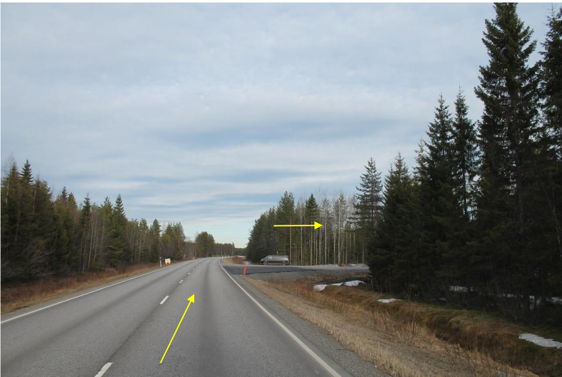
Pos 23/Pic 34. Site entrance. Turning from Road 27 toward Murtomäki site area. https://goo.gl/maps/cJiUoRQA4bXGdQZQ7 Site entrance to be constructed according to turbines suppliers specifications.
