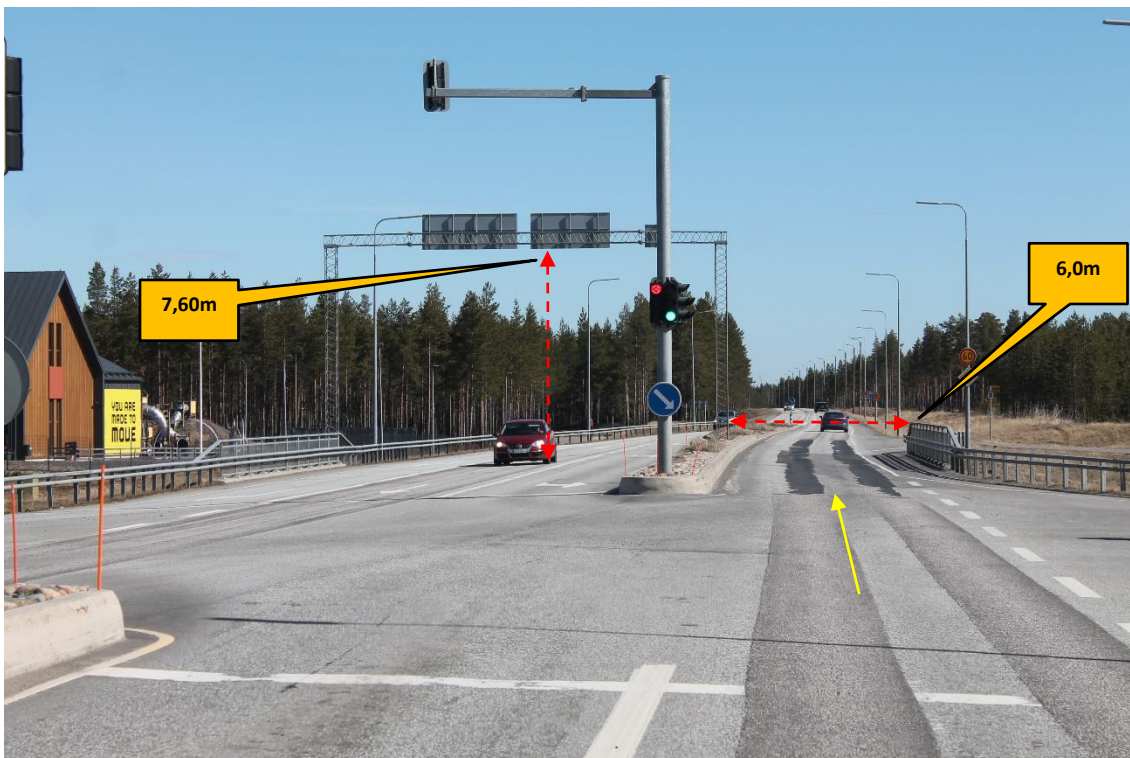
Pos 3/Pic 6. Road 8. Modifications: N/A. Height of the rail is 1,10m.
