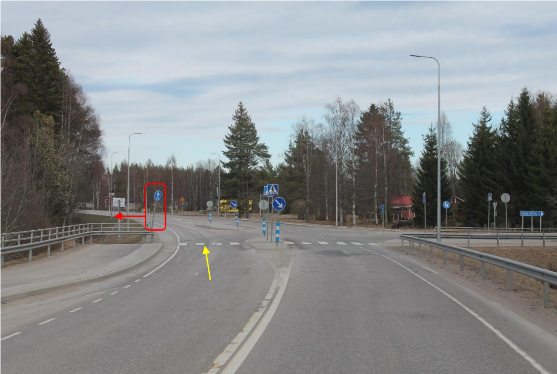
Pos 22/Pic 33. Road 27 in Haapajärvi. https://goo.gl/maps/AQ9DrfitjNp9Cs8v9 Marked sign need to be removed.
