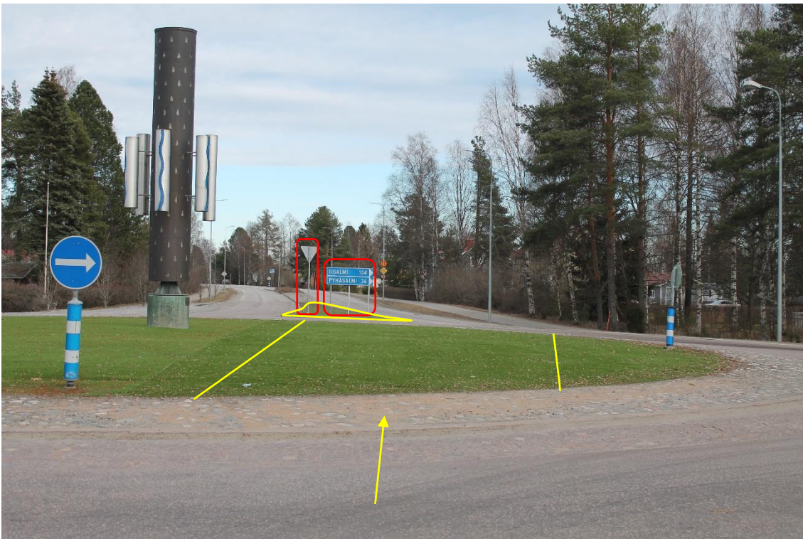
Pos 20/Pic 30. Road 27 in Haapajärvi. Need to build road thru roundabout. Marked areas need to be filled and drivable. Marked signs need to be removed.
