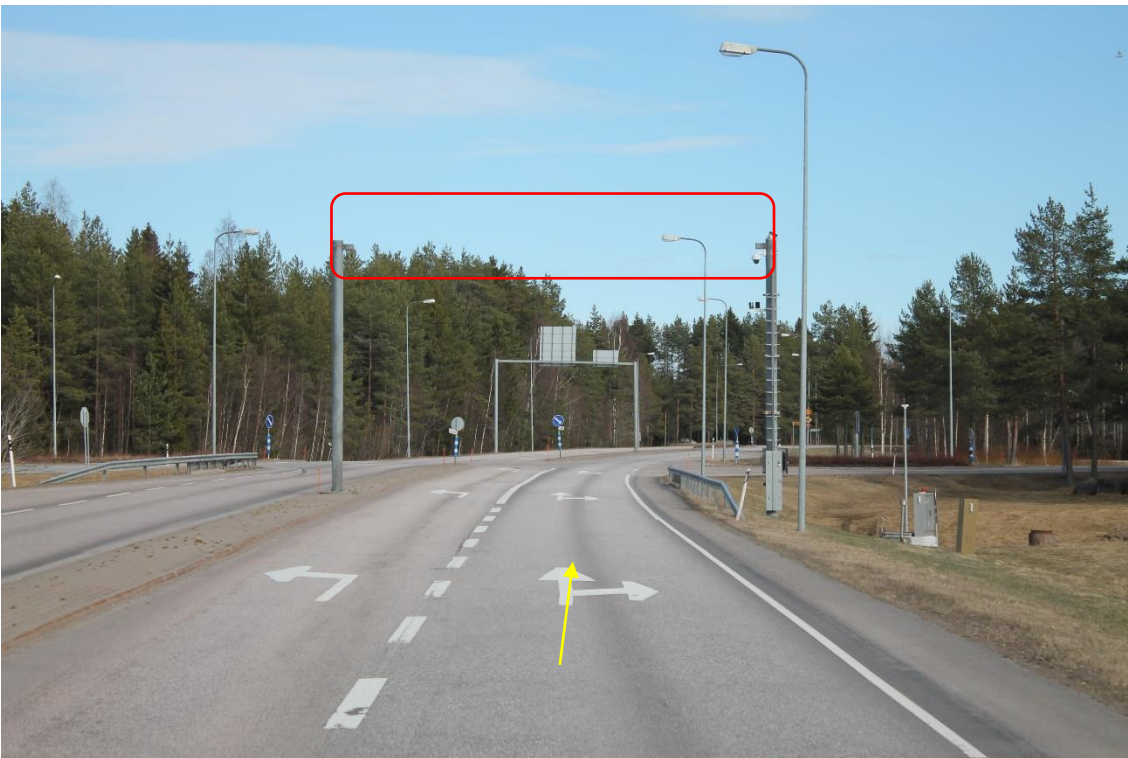
Pos 5/Pic 10. Road 27 in Alavieska. https://goo.gl/maps/qwZE6KPTHdZaPBt59 Marked portal (missing) need to be removed.
