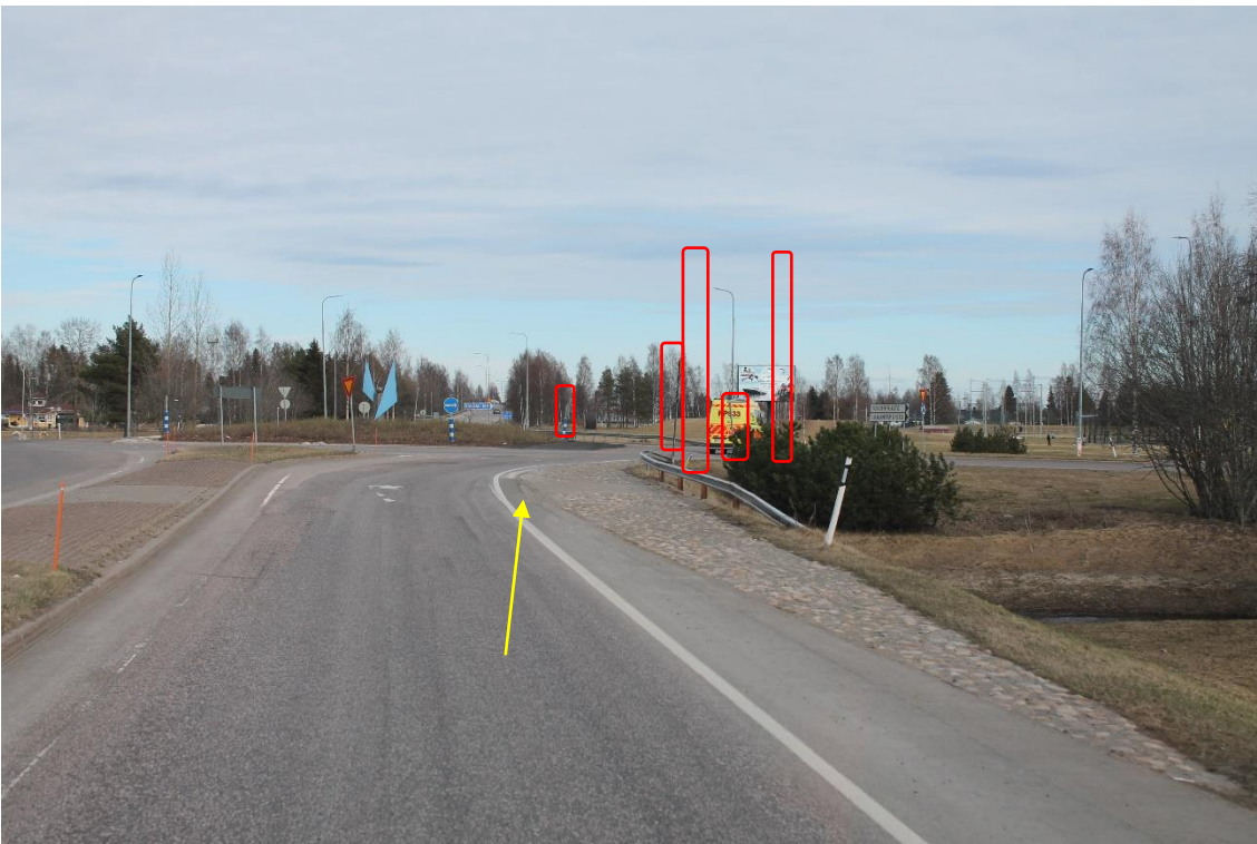
Pos 8/Pic 14. Second roundabout on Road 27. https://goo.gl/maps/MSQUoRtCQnoKuMHTA Continue straight on road 27. Marked signs and lamp posts 2pcs (missing) need to be removed.
