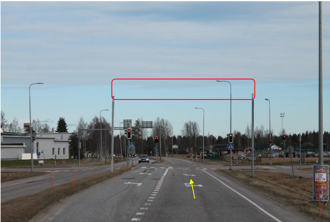
Pos 16/Pic 25. Road 27 in Nivala. https://goo.gl/maps/koozJ1AvfJ2ir4Hi9 Marked portal need to be removed.
