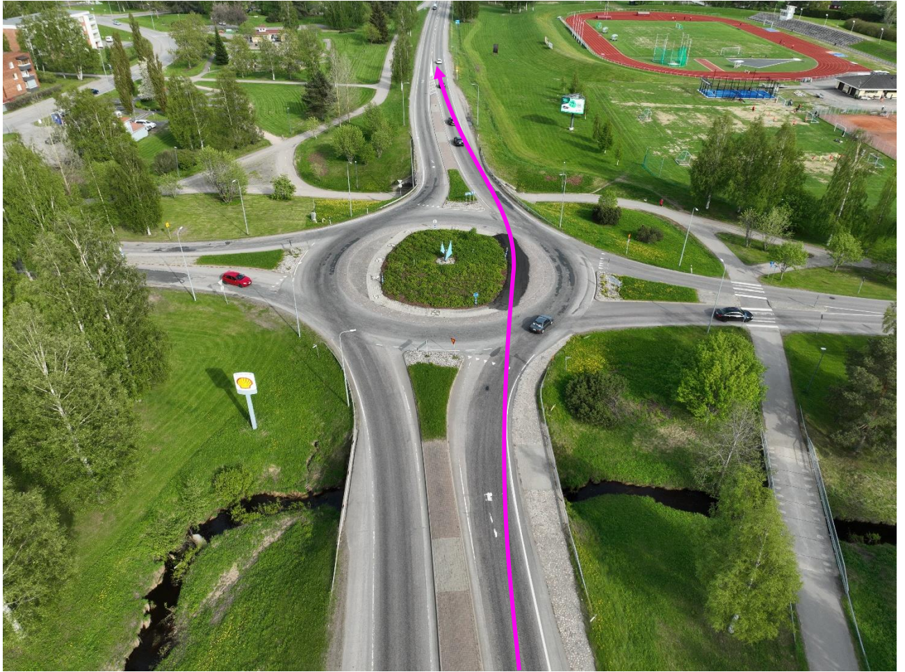
Second roundabout in Ylivieska has been modified in center part by driveable extension and removals of light poles.
