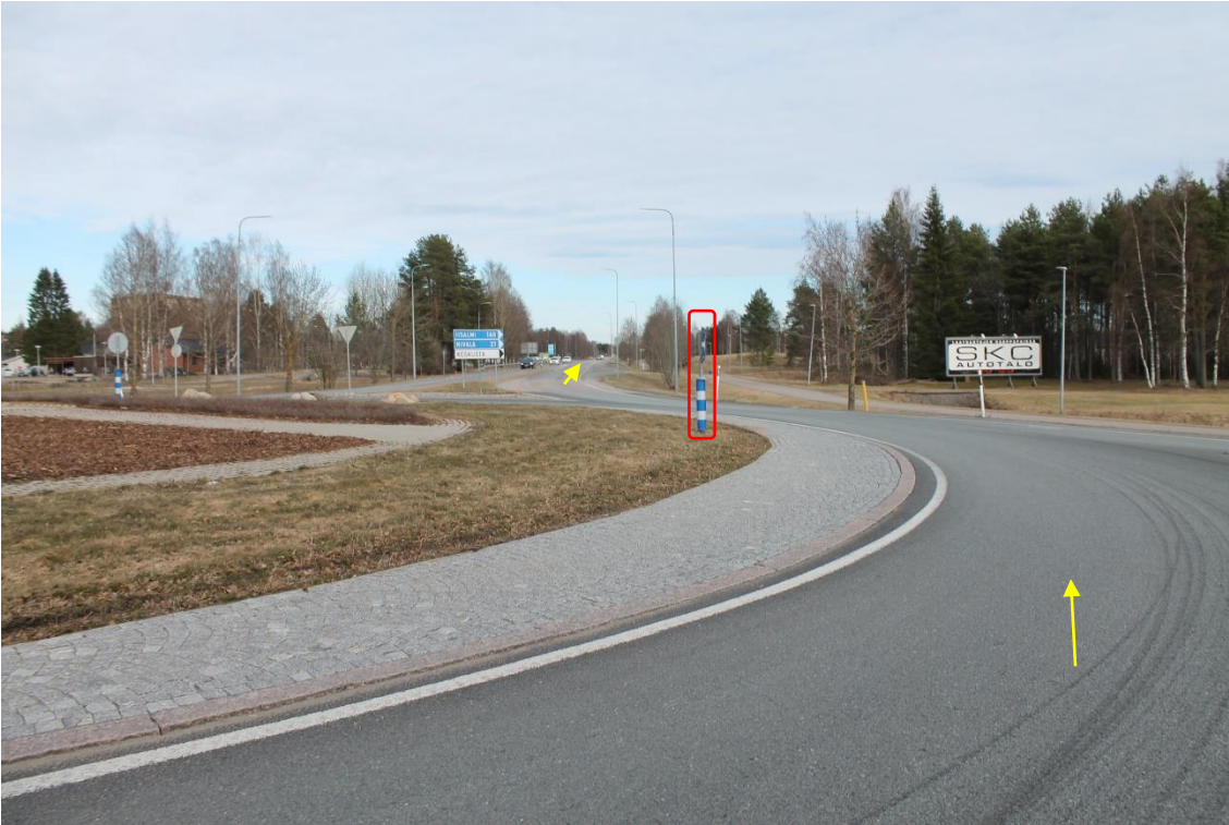
Pos 7/Pic 13. First roundabout on Road 27. Continue straight on road 27. Marked sign need to be removed.
